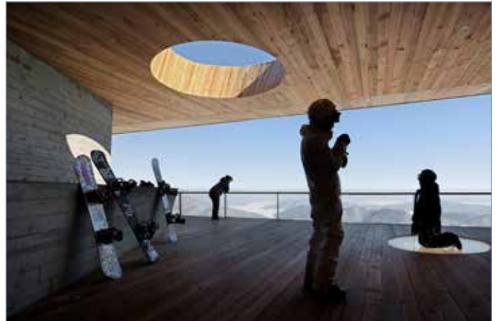
▲ Two circular openings cut through the red cedar ceiling and floor. While the top hole allows sunlight and snowflakes to enter, the floor window gives visitors a chance to observe the skiing activities below.
