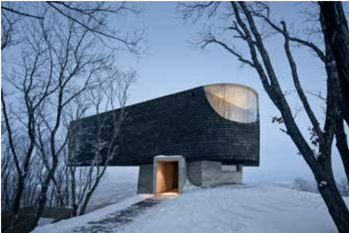
▲ Inspired by a piece of leaf floating on water, the boomerang-shaped structure's location was selected due to its unobstructed view of the surrounding area, and its minimal impact to the forest.
